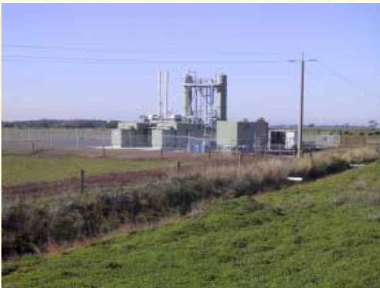
Werribee biomass (sewage methane) plant
