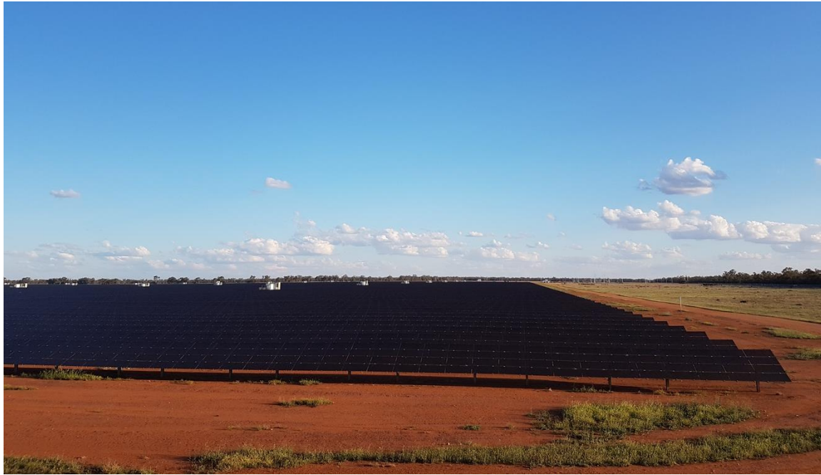
Figure 5.1 Nyngan Solar plant
